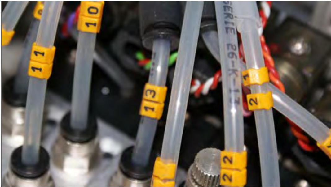
Fig. 3.2.3: LHS – Marking of the tubes
