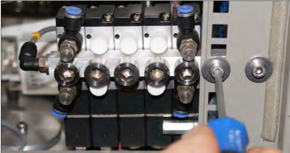
Fig. 3.2.1: LHS – Removal of the valve block
