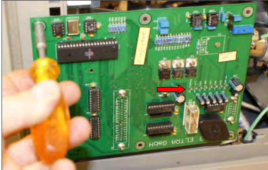
Fig. 1.6: RHS - Main bord (voltage measuring points marked by red arrow)
