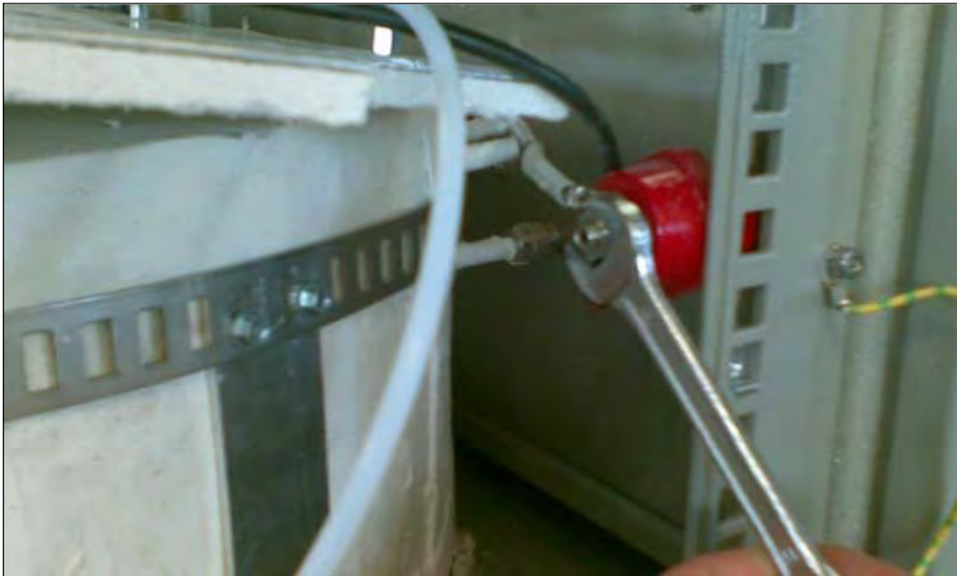
Fig. 3.16.5: LHS/RHS – Disconnecting the furnace and electrical support wires
